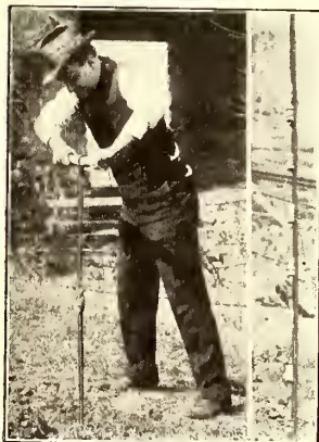
PREPARING TO BLAST A POLE HOLE; VIEW OF DYNAMITE STICK
